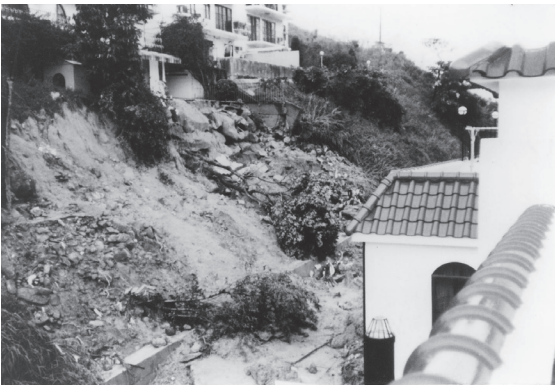
Figure 5. General view of failure - case 2
